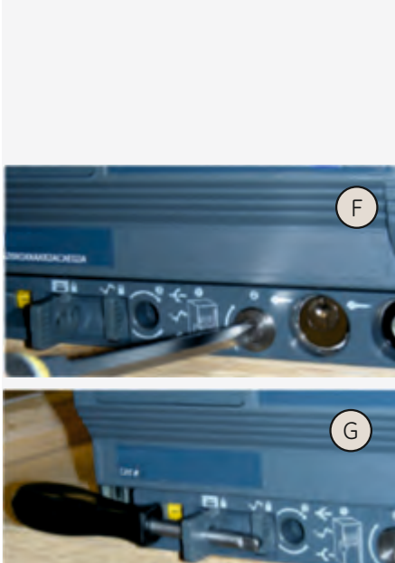
Fig. F: Attempting to open the racking handle aperture. Fig. G: Blocked security locking bar. Fig. H: The Closes button used to switch the breaker ON. Fig. I: Depressing the "OFF" and removing the Key.
