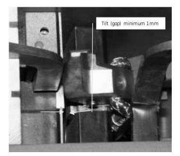
Fig. 46 Inspection of the main contacts' tilt
