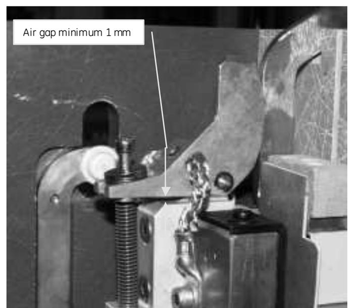
Fig. 47 Inspection of the arcing contact's air gap
