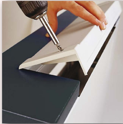
Quick mounting of cable-entry panel
